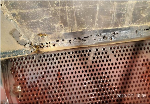
HPH-5 plate welding joint
