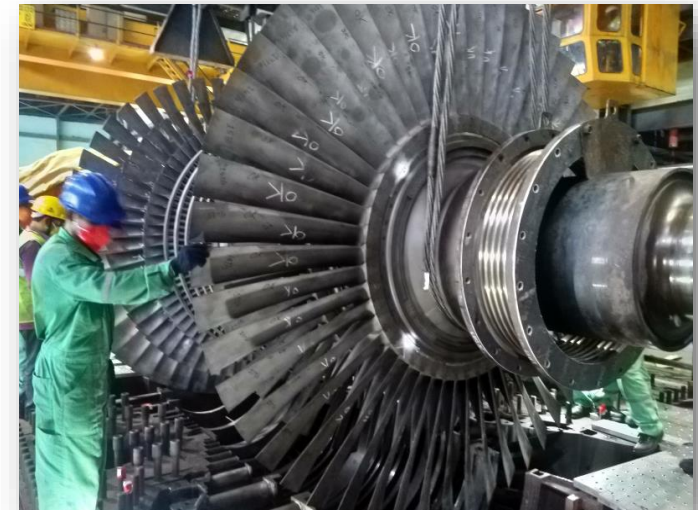
Servicing LP turbine
